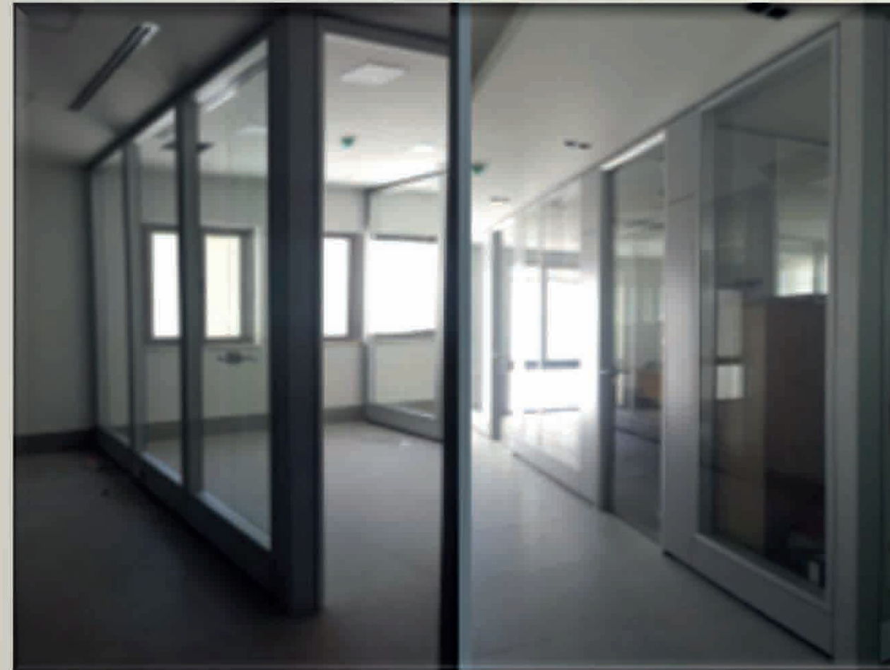
Client: Miqdadi Project Job: Office partitions- Amman/Jordan
